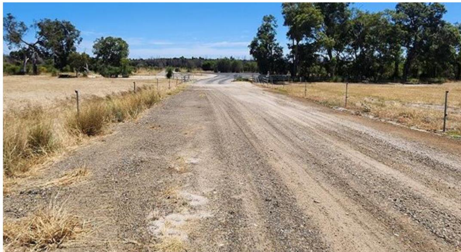
CAUSEWAY NORTHBOUND (SHIRE OF WAROONA)
