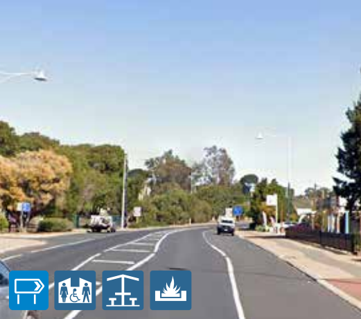
Southbound South Western Hwy - install large blue directional sign 100m prior to park entrance
