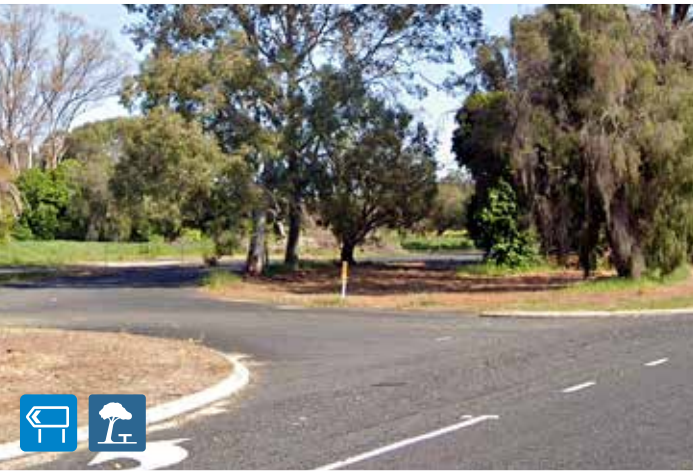
Old Coast Rd Rest Area - This rest area has everything including slip lanes, but has no advance warning or directional signs
