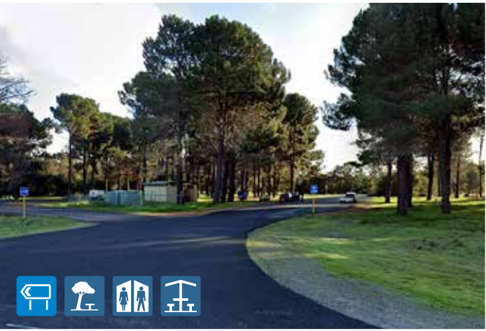
John Tognela Rest Area, Forrest Hwy - This rest area is well signed with advance warning and directional signs.
