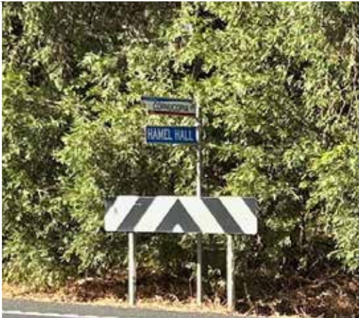
Overgrown fingerboard signs at South Western Hwy/ Cornucopia St
