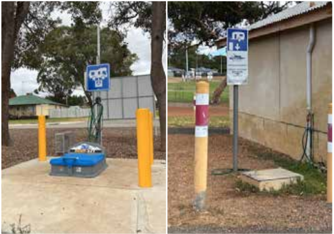
Waroona Railside and Showgrounds RV Dump Points. Improve signage at the Showgrounds dump point
