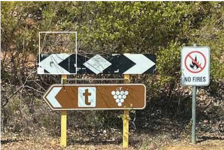
Some advance warning and directional signs at Waroona Dam are overgrown.
