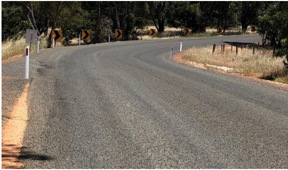
Photo 21: Southern Estuary Road reconstruction
