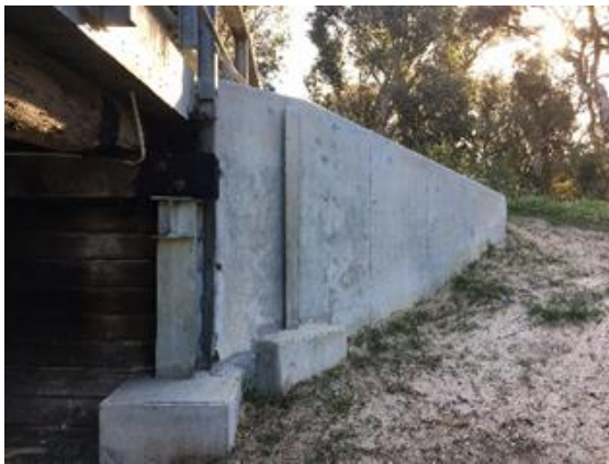
Photo 22: Repairs to Lake Clifton Road bridge
