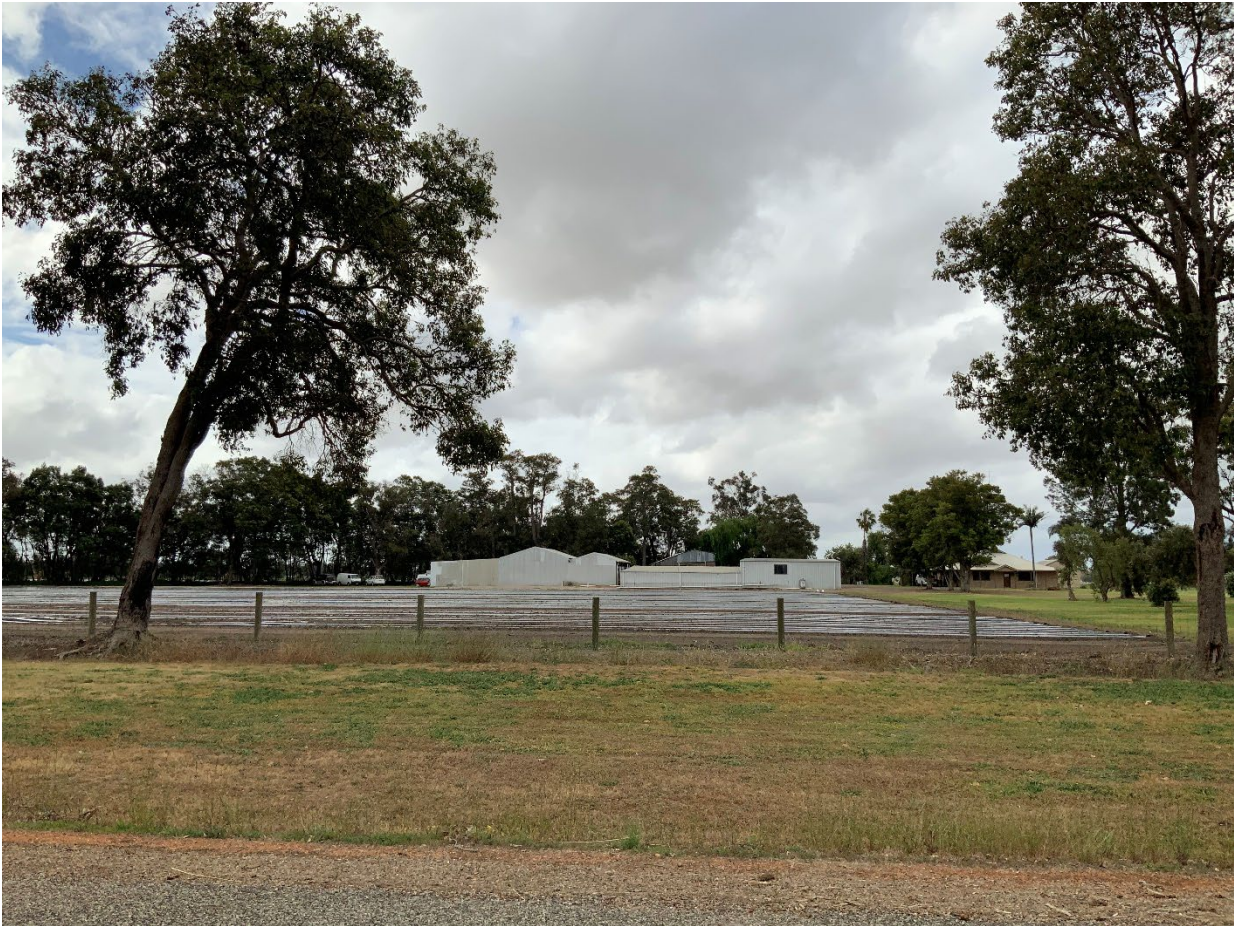
View of the workforce accommodation from McClure Road
