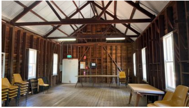
Interior view looking south.
