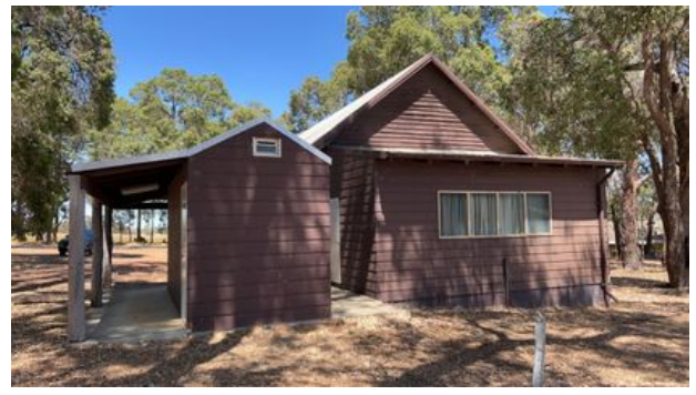
North elevation. Toilet block at left.
