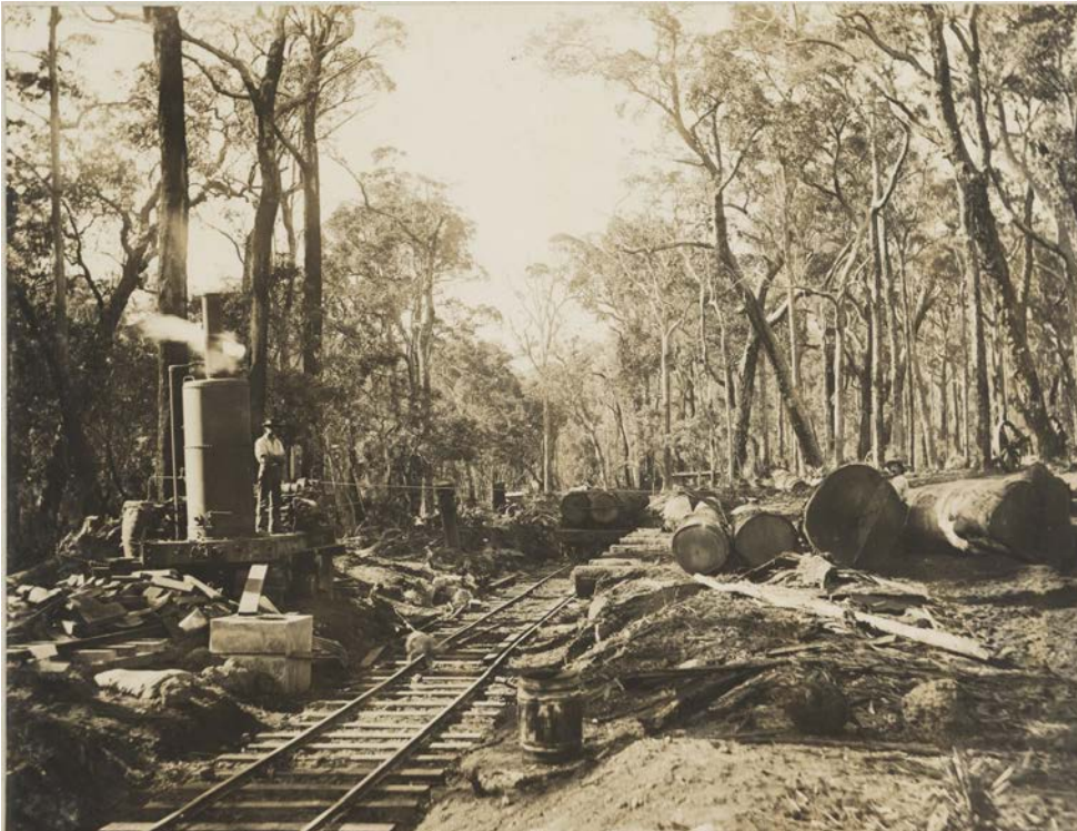
Figure 12. A steam crab winch at a log landing at Waroona, c. 1900. (SLWA 1458B/6a)
