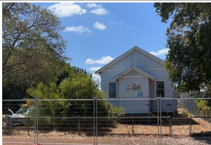
February 2023, prior to demolition.
