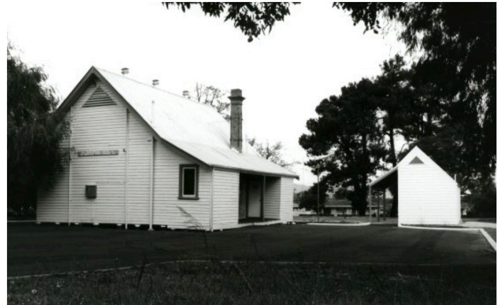
Figure 20. Drakesbrook Primary School before it was destroyed by fire.
