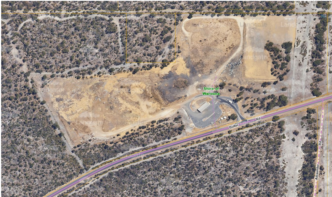
Figure 6: Overview of the Buller Road Waste Facility.
