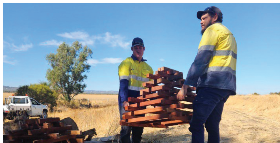
Image: Fish Hotels delivered to site ready for installation along the Harvey River.
