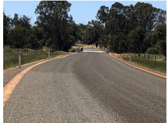
Photo 19: Coronation Road reconstruction
