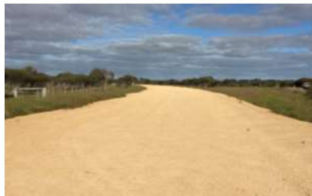
Dorsett Road realignment to sub-base stage
