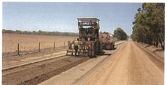
Contracts from Western Stabilisers applying the cement stabilisation to Coronation Road.
